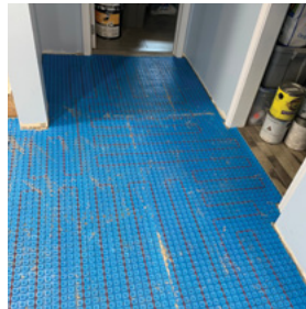
Basement with Prodeso Membrane
